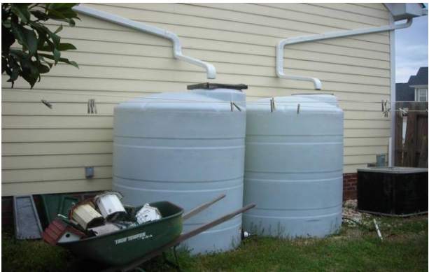
Rain Barrels with Roof Drains
